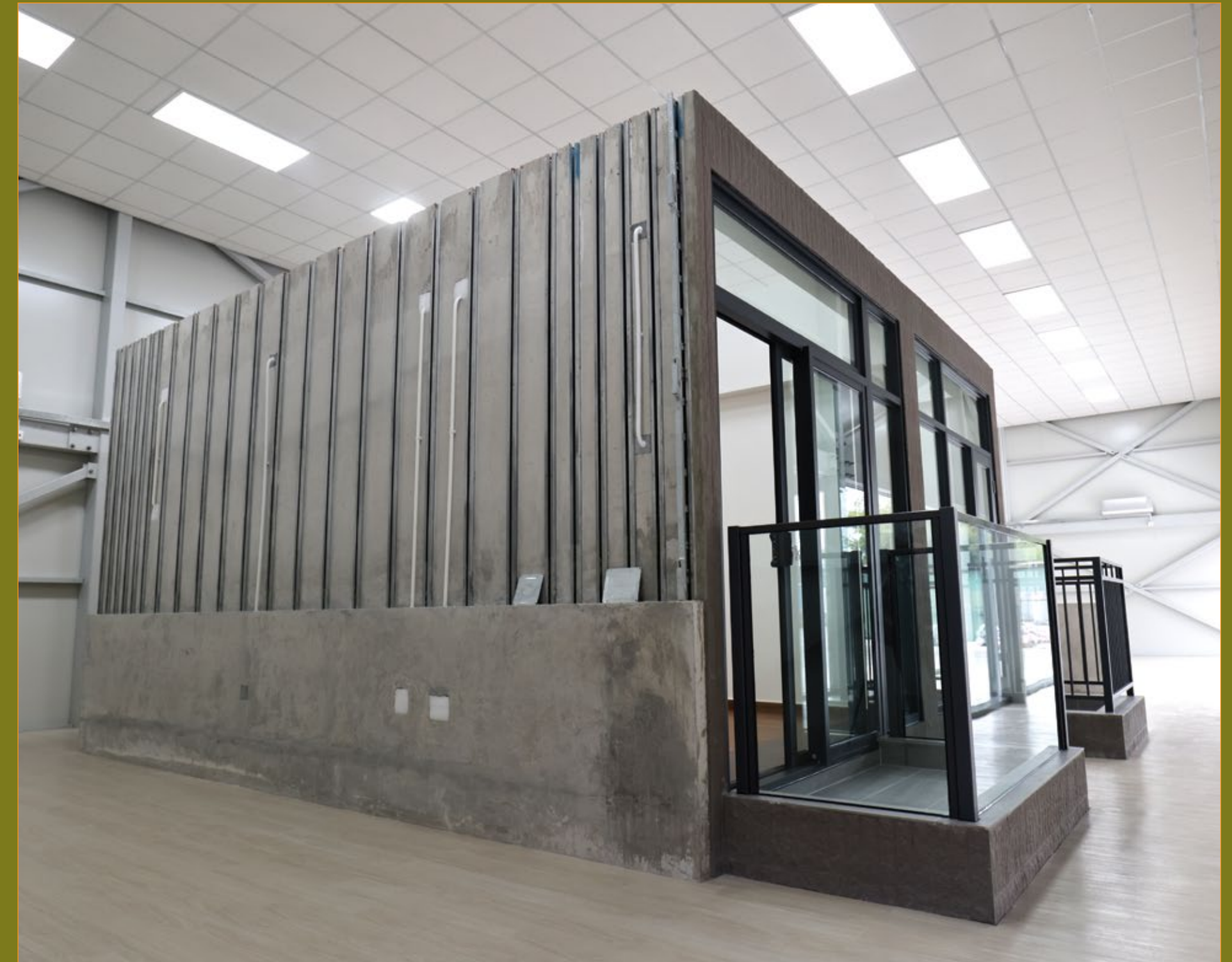
Above: Show flat built with 'Chun Wo Concrete MiC Systems' Below: Patented 'Wall Connection System'
